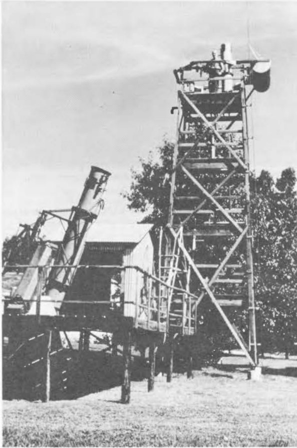
Figure 10. Dr. Everhart's Wormwood Hill Observatory in Connecticut. The 11 \frac{1}{2} -inch reflector is mounted on a 30-foot tower to provide a good horizon above the trees. It stands on concrete piers. The telescope is covered by the round, corrugated metal piece on the right side of the platform; and there is also a lightning rod.
